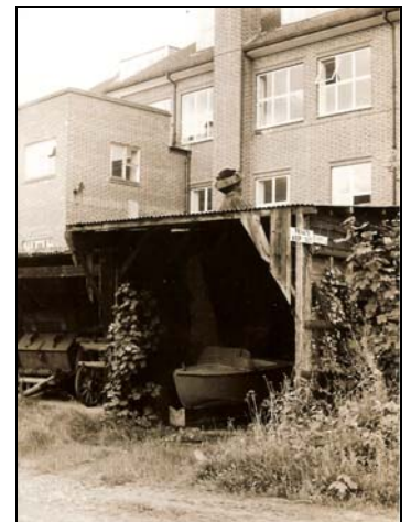
The steam-roller's shed – still with chimney fitted into the roof – at Hundreds Farm, Westgate
